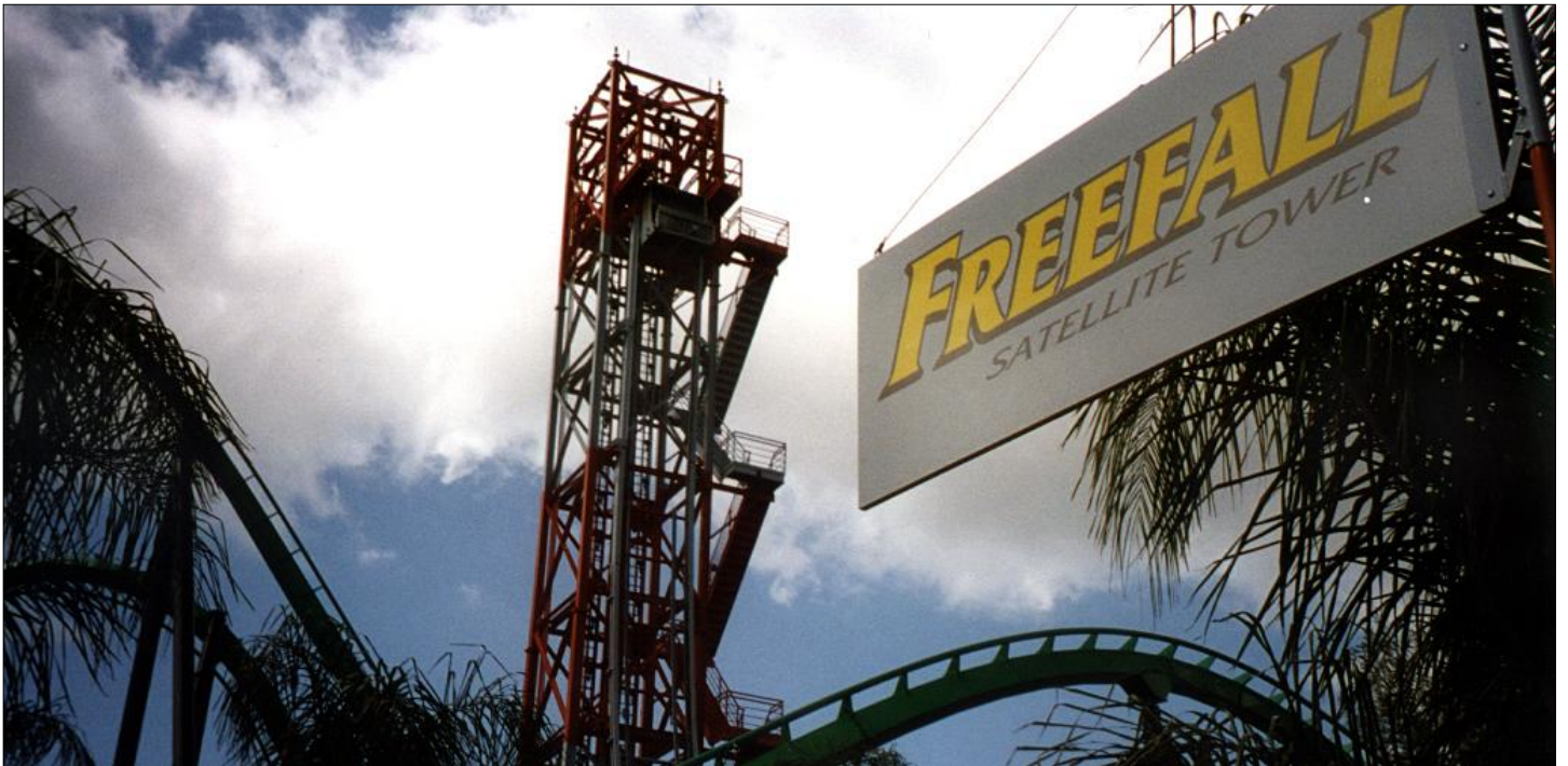
Freefall satellite tower, where the ride cage drops vertically on the outside of the tower after going up the inside.
