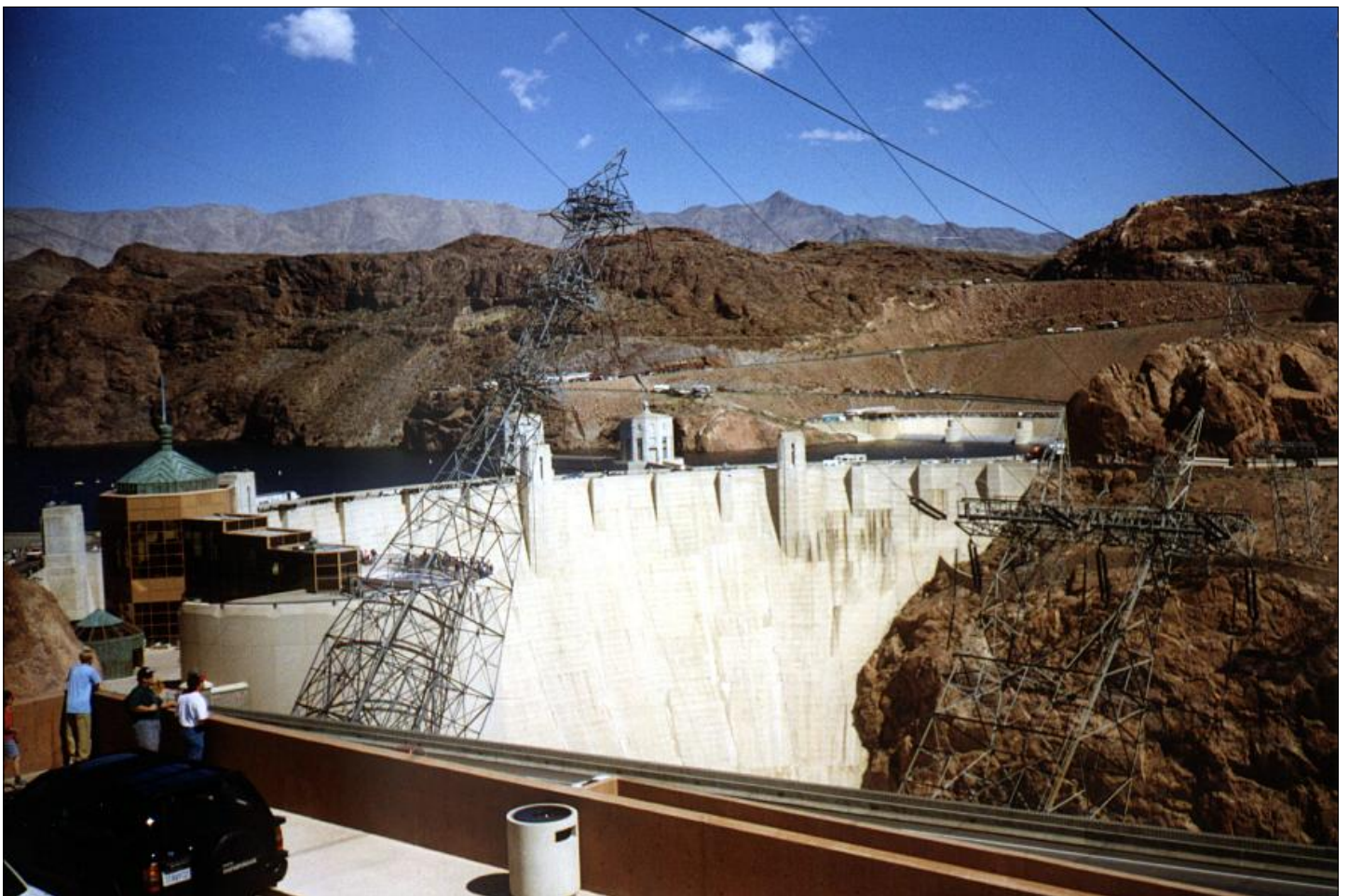
Hoover Dam with the leaning pylons that bring generated electricity up from the powerhouse and out of the canyon.
