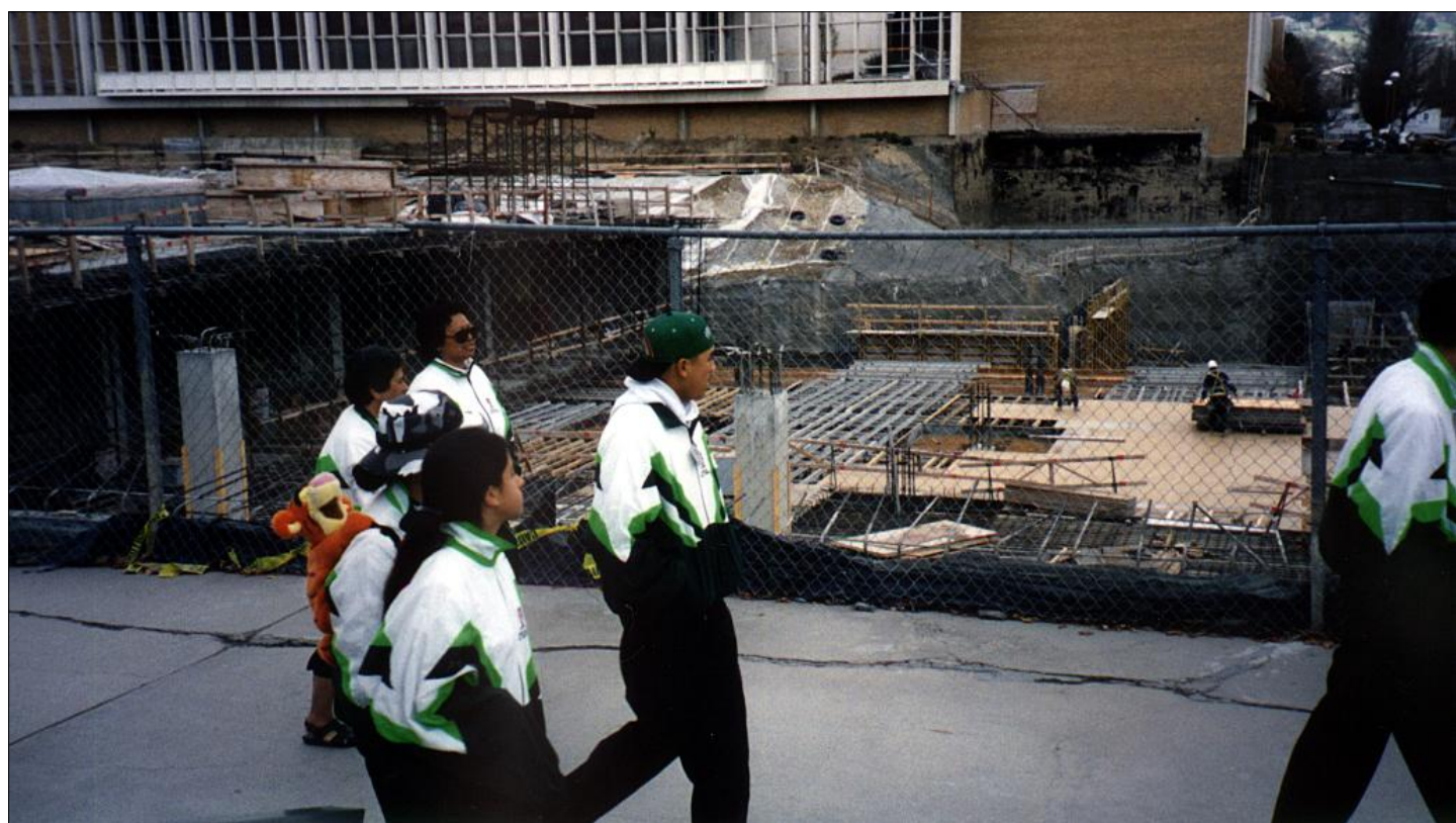
Robyn, Wynel, Piata and Te Whainoa head past a construction area at BYU. Being built is a four-story public genealogical library, all underground. The roof will become part of the campus lawn. The structure will become the largest public genealogical library in the world. Building below ground level enables better control of building temperatures for the safe storage of genealogical files.
