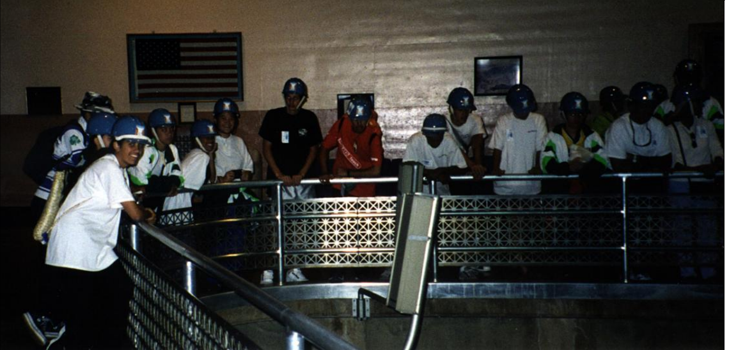
(Top and Above) The group looking over the balcony over the generators that supply Las Vegas and Los Angeles with all their electrical needs.
