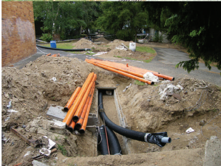
After 45 years of operation it was time to replace all of the underground pipes that carry heated water to the school buildings. The work was completed three weeks into Term 1.
